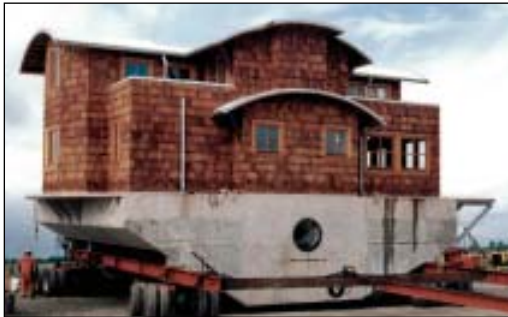
The home's foundation includes an underwater observation room with a porthole for viewing local marine life.
