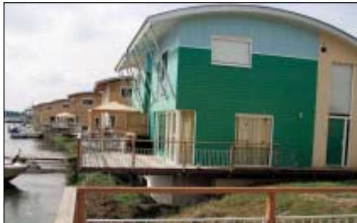
"Amphibious homes" built by Dutch construction company Dura Vermeer start at 260,000 euros (approximatel $347,000). The foundations, which rest on the bank, are hollow concrete cubes designed to float, and power, water, and waste are delivered through flexible conduits that accommodate movement whenever the Maas River floods.
