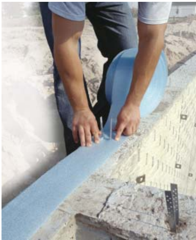
STYROFOAM SILL SEAL GASKET
